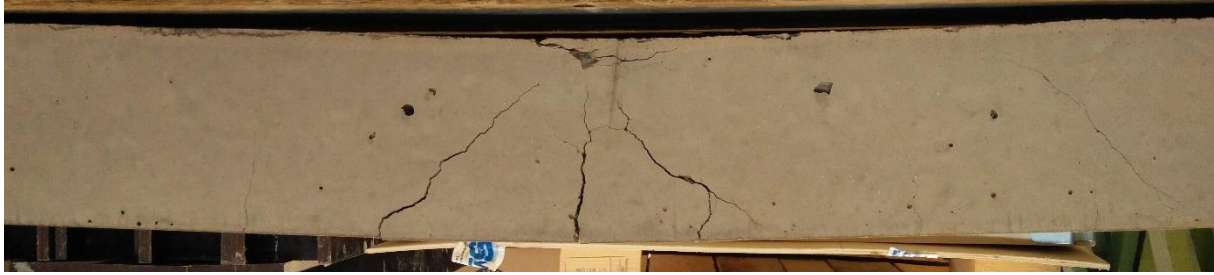
Figure 6.24 Crack pattern displaying a horizontal crushing crack, shear cracks and bending cracks. Photo by Erla Sara Svavarsdóttir.
