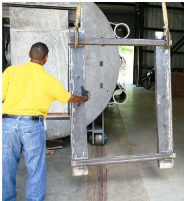
Figure 2 Photograph of blast side fixture about to be assembled over the previously placed concrete slab (directly behind technician).
